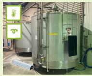
Exposed metal on older vats, hot water cylinders and pipes: wraps can be installed to save energy.
